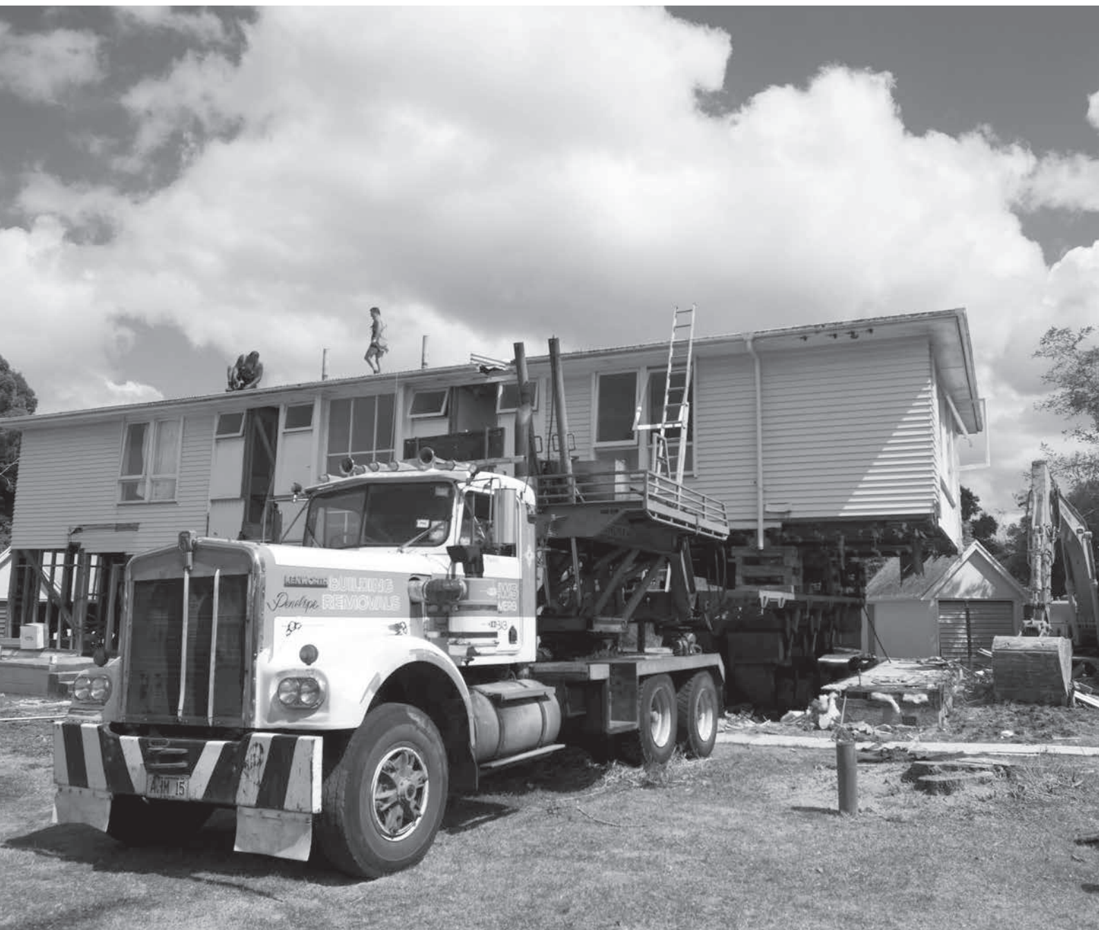
State houses on Haverstock Rd, Sandringham, Auckland, that are being removed by Housing New Zealand.
